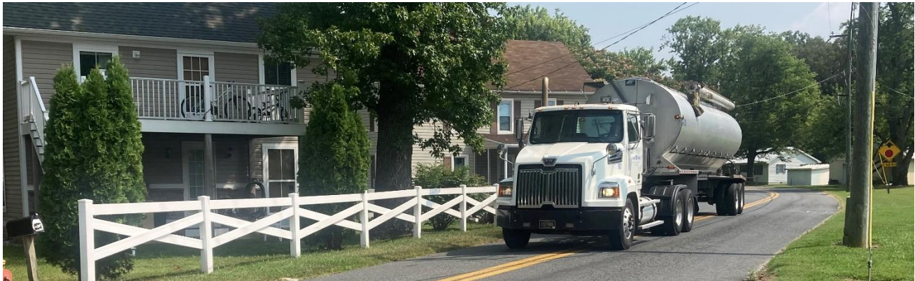
Figure 8: Narrow Shoulders and Lane Encroachment in Delmar
