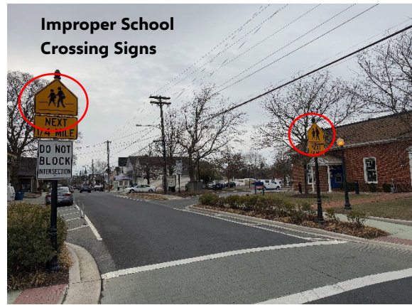
Figure 5.15: Improper School Crossing Signs SB MD 272
