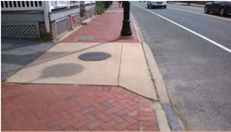
Example of level sidewalk with driveway apron using sloped edge only. Most driveways on Main Street stand out to drivers and pedestrians through the use of contrasting concrete pavement.
