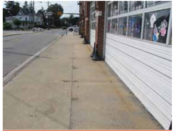
Former fire station driveway is sloped, making it uncomfortable to walk on and not ADA compliant.
