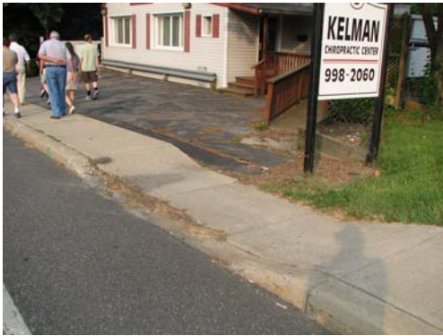
Figure 6: Sidewalk slope issue on OCT
