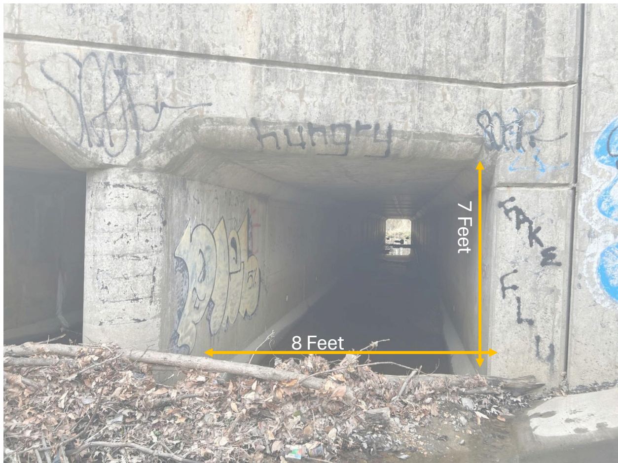
Figure 10: The Entrance to the Rocky Run Culvert Cell
