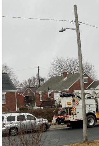
New Street Light Installed in Collins Park, February 2025
