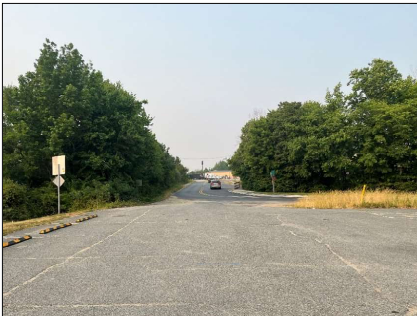
Figure 3-2: I-95 at MD 279 Park and Ride Facility
