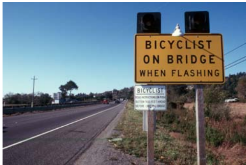
Example bridge bicycle detection signage
