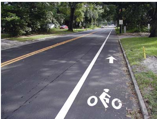
A shoulder with pavement markings to accommodate bicyclists.
