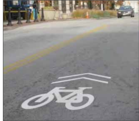
Exhibit 28: Shared-use lane markings, known as sharrows, were installed in late 2010 along Market Street.
