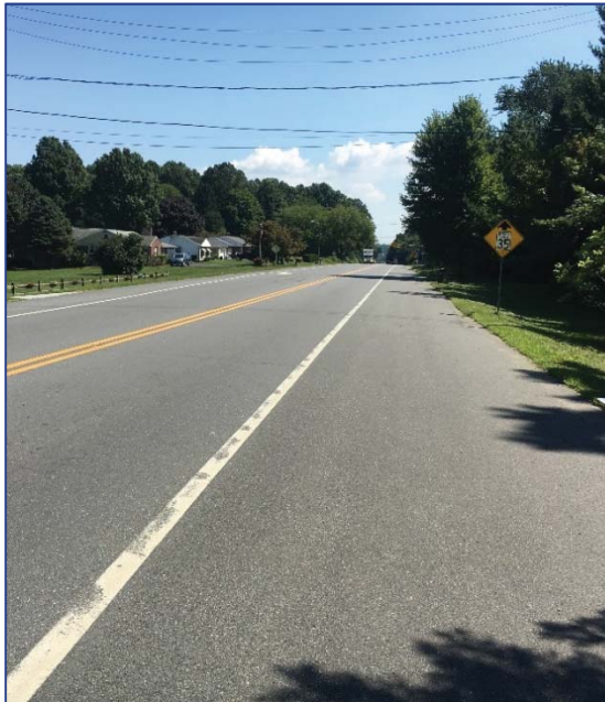
Figure 6 SR 41 SB VWS site, south of VFW Post 5892 looking southbound.
