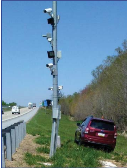
Figure 3: SR 1 VWS Pole
