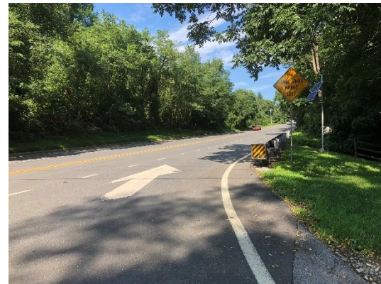
Photo 4: Southbound Hickory Spring Rd corner sight distance looking right onto SR 48 (beyond "stop line")
