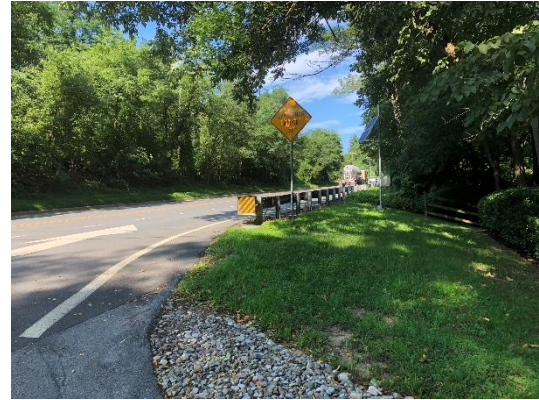
Photo 2: Southbound Hickory Spring Rd corner sight distance looking right onto SR 48 (from "stop line")
