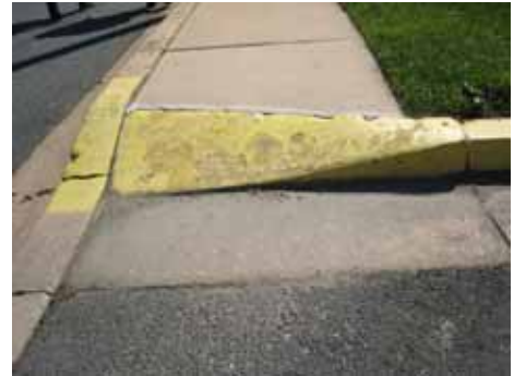
On Booth Street curb cuts are too steep to accommodate the disabled.
