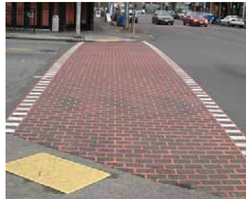
A textured and/or colored crosswalk is an aesthetic treatment used to make a crosswalk surface more visually attractive.
