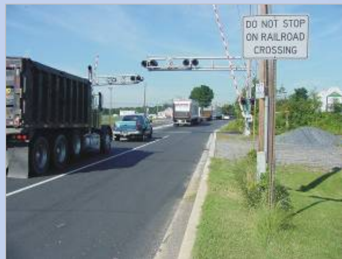
Westbound Boyds Corner Road at US 301
