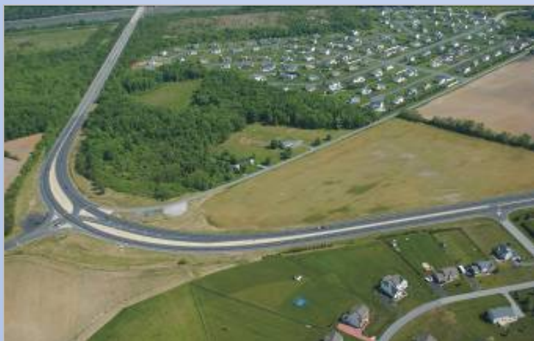
Sharp Curve South of Summit Bridge
