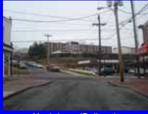
Neckdown (Bulbout) Maryland Ave @ Cedar St
