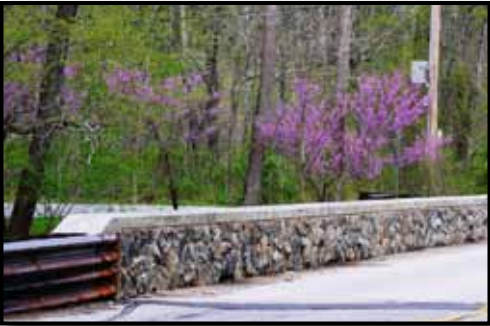
Figure D-5. Concrete bridge abutment with stone veneer and weathering steel guardrails at entrance to Spring Valley.
