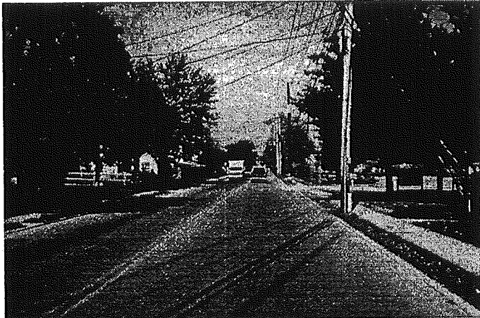
Chapel Street looking northbound
