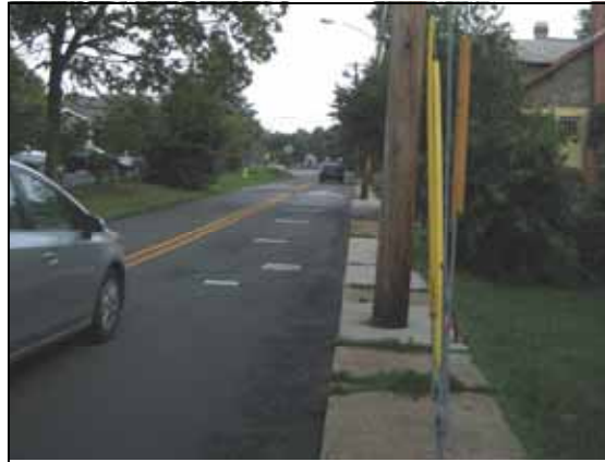
Utility poles and guy wires impede pedestrian movement along the narrow sidewalk.
