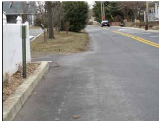
Looking northbound on Locust Lane, where southbound lane widens mid-block.
