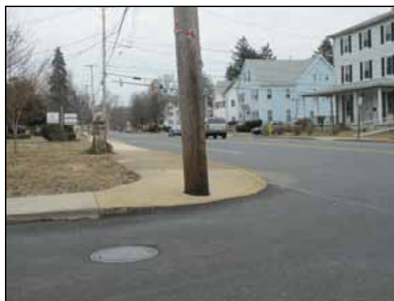
Locust Lane at Main Street lacks striping for a pedestrian crosswalk.
