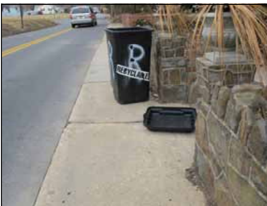
Obstacles impede pedestrian movement and force sidewalk users into the street.
