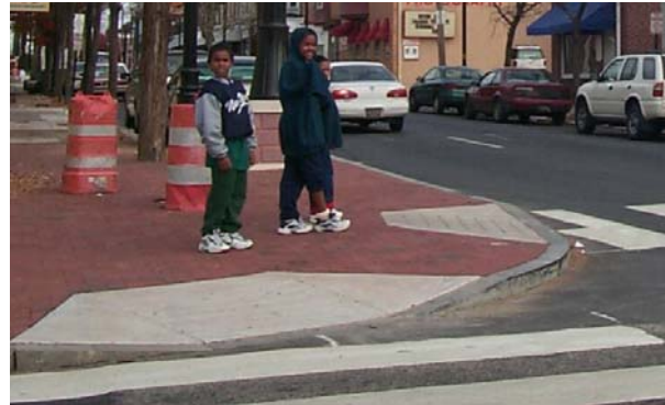
This well-designed intersection has two curb ramps direct pedestrians in the direction of travel for each crosswalk. Different colored/textured pavement help those with sight impairments.
