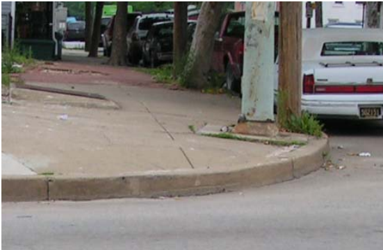
Lack of curb ramp hinders travel by persons with disabilities, parents with strollers, children and the elderly.
