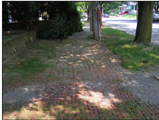
Sidewalk along Shallcross Avenue in Wilmington
