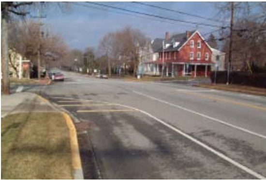
7Q - Existing Configuration Looking North
