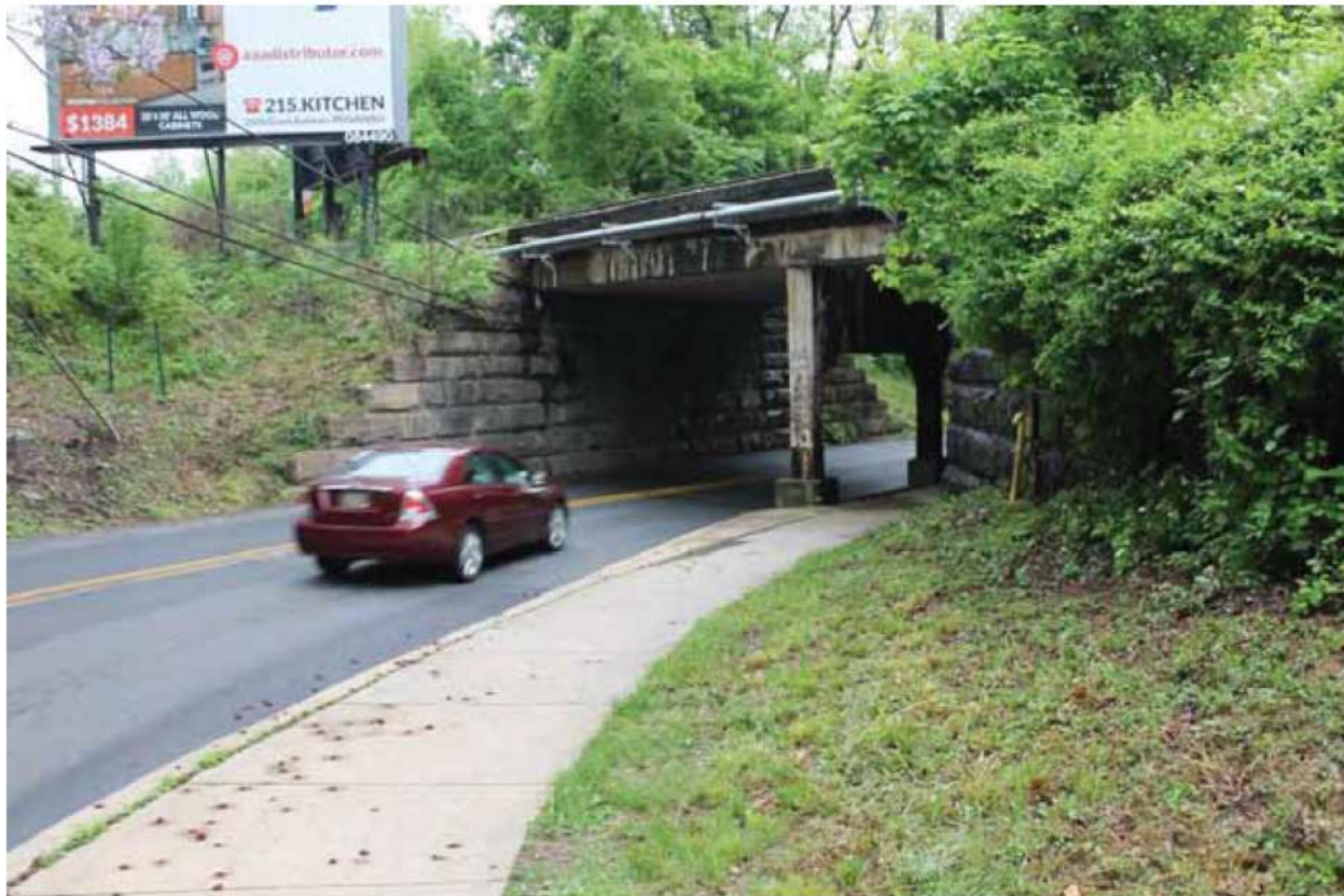
Figure 11: Approach to the railroad bridge underpass on West 18 th Street from the north side of the bridge. Limited sight lines and a narrow passage should be addressed by alerting users with pavement markings, signage, and other methods.
