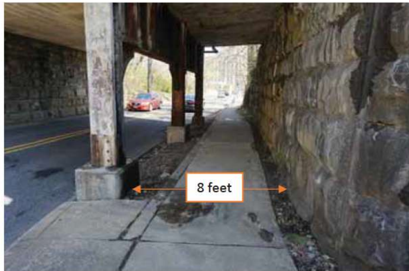
Figure 10: Existing sidewalk under railroad bridge along West 18 th Street, looking south/east; clearance between pier and wall measures 8 feet.
